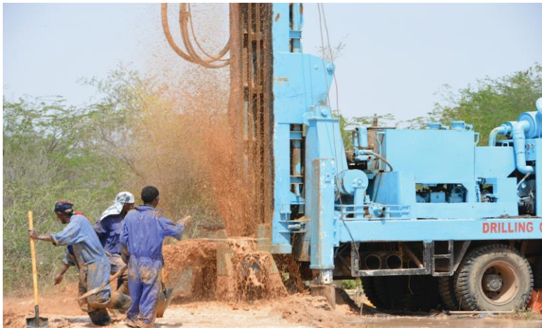
Borehole drilling in progress
